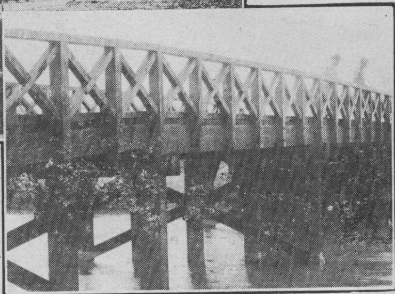
橋架木河沙之內段江浙：上 Above—A Timber Bridge—Chekiang Section.
