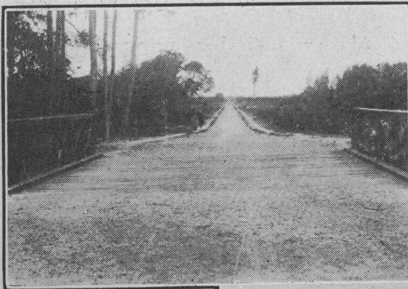
Above—Broken Stone Pavement with Shell Surfacing—Chekiang Section.
