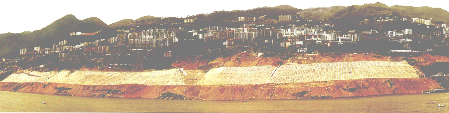
库区新城 (巫山) A new city by the reservoir (Wushan County)
