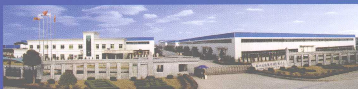
临平厂区外景 Outdoor scene of Linping factory
