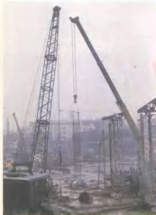
该局工程公司正在进行基础桩基施工 The Engineering Co. of the Bureau is constructing pile foundation
