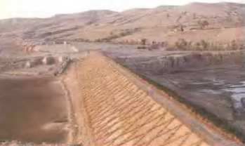
内蒙古境内有草场护坡的骨干坝 One of the key dams in Inner Mongolia Autonomous Region. The slope is protected by grasses.
