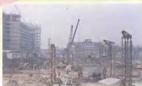
该局工程公司承建的郑州市金博大工程工地 The construction site of Jinba Great City in Zhengzhou which is built by the Engineering Co.
