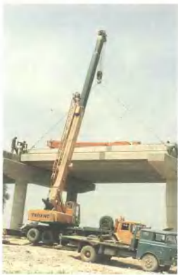
文源工程公司在开封黄河公路大桥施工 Wenyuan Engineering Co. is constructing Kaifeng Yellow River Highway Bridge.
