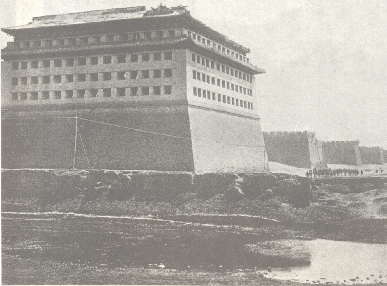
图1-9 Corner Tower of the City Wall 北京城角楼
