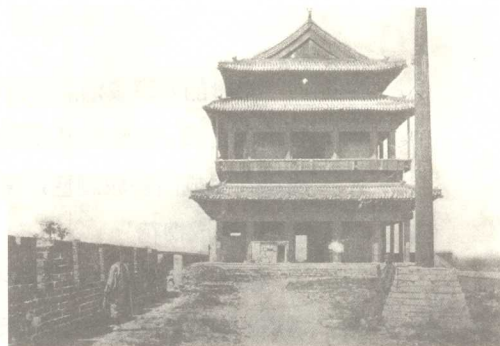
图1-4 Photo of Side View of the Top of chongwenmen 崇文门顶部
