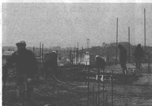
(c) 柱梁板一次浇筑
