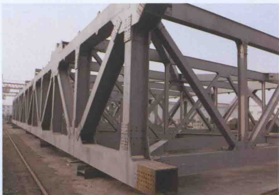
↑ 钢桁梁厂内组拼
