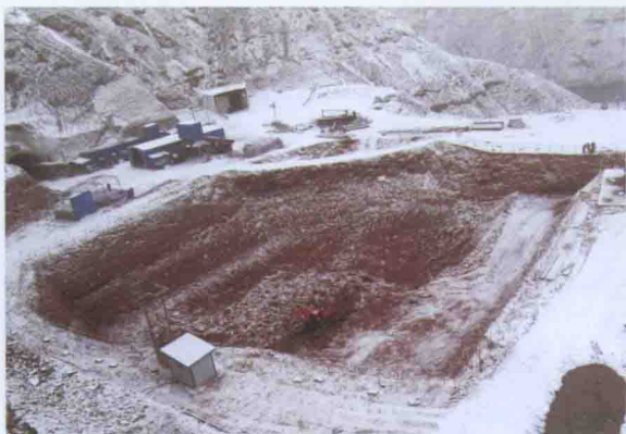
↑ 锚碇基坑开挖
