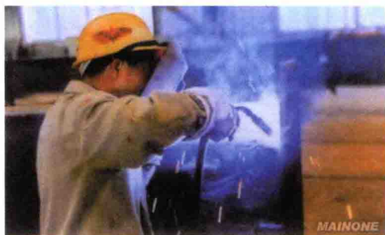
Gas metal arc welding (GMAW)
