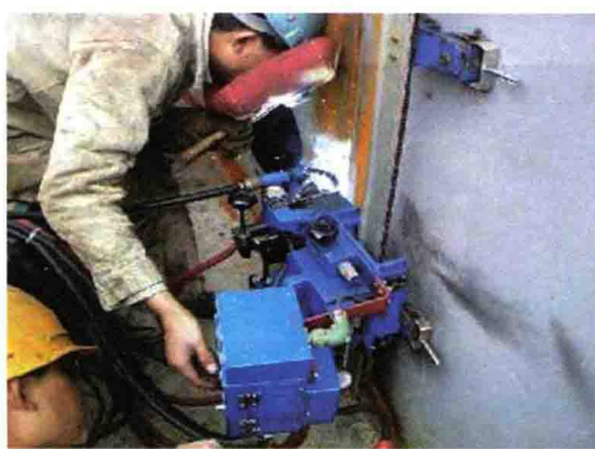
Electrogas welding (EGW)
