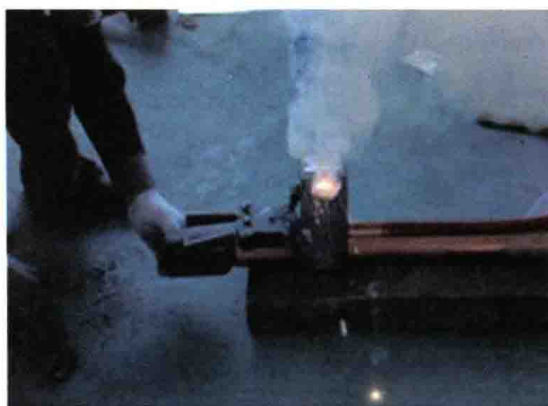
Thermit welding (TW)
