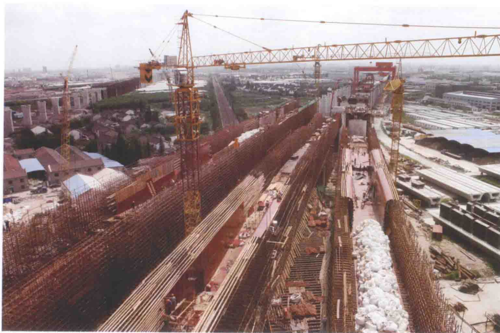
◀ “三角区”现浇连续梁施工
