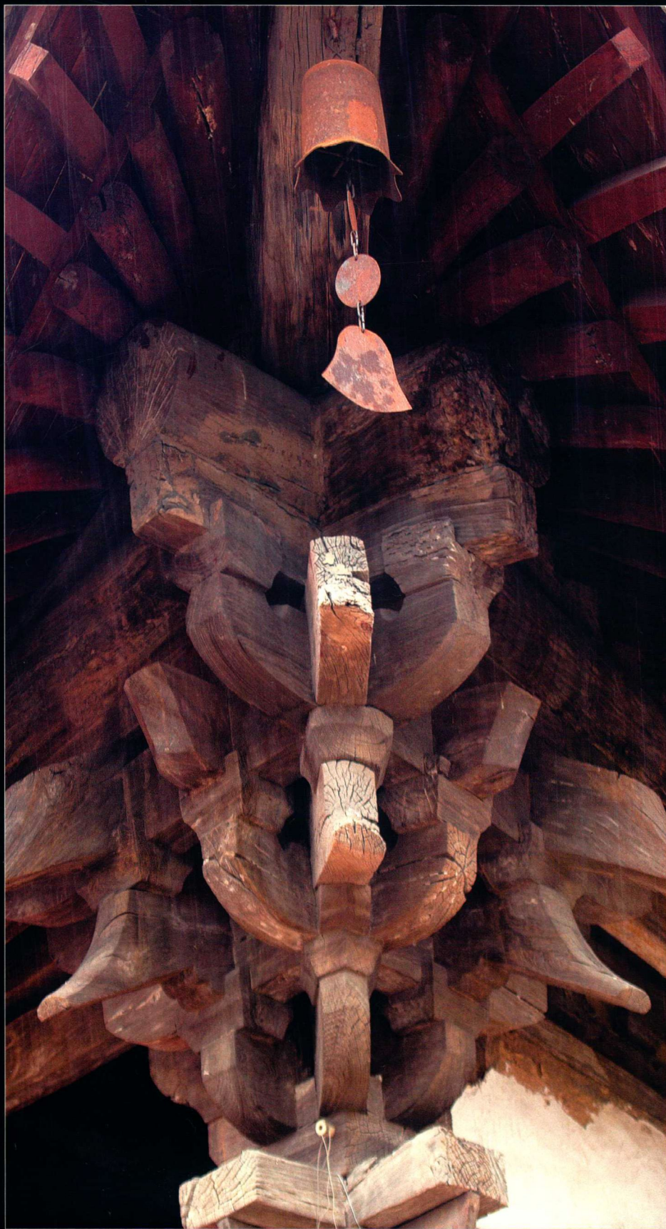
雨中中殿檐角 Eaves corner of the Mid Hall
