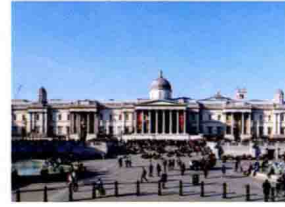
4. National Gallery William Wilkins (original), E. M. Barry (interior) Trafalgar Square, Westminster 1838 (p. 24)
