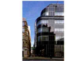
12. Daily Express Building Ellis and Clark, Owen Williams Fleet Street, City 1932 (p. 42)
