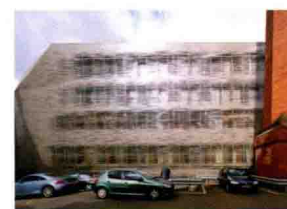
50. Town Hall Hotel & Apartments RARE architecture Patriot Square, Tower Hamlets 2010 (p. 114)
